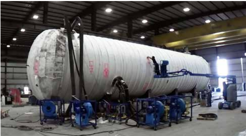
Figure 2: Seven high-velocity gas burners line the base of a 621,000-pound pressure vessel in Central Texas as insulation wrap nears completion. Gulf Coast Combustion documented the full PWHT cycle on this job via time lapse footage. (Courtesy: GCC)
