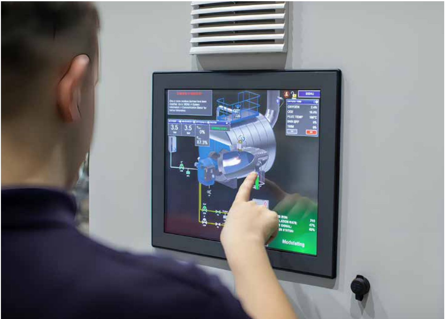
Combustion control panels can now communicate with site-wide automation systems using standard industrial communication architectures. (Courtesy: Dunphy Combustion Limited)
