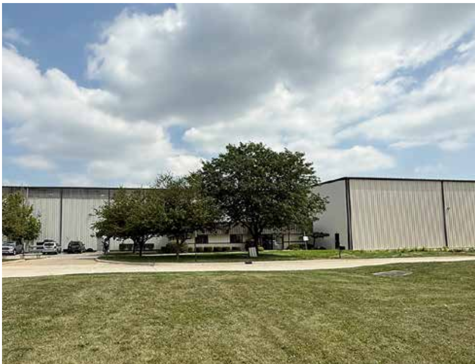
Advanced Heat Treat Corp. recently expanded its Michigan location to accommodate the company's growing needs. (Courtesy: Advanced Heat Treat Corp.)
