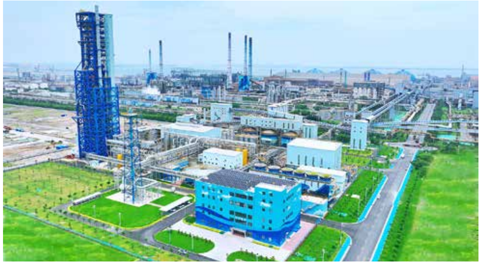
The sustainable hydrogen-based 1,000,000 metric tons/year Energiron Direct Reduction (DR) plant demonstrated the nominal production of DRI, reducing carbon dioxide emissions and marking a significant step in the green steel industry. (Courtesy: Tenova)
