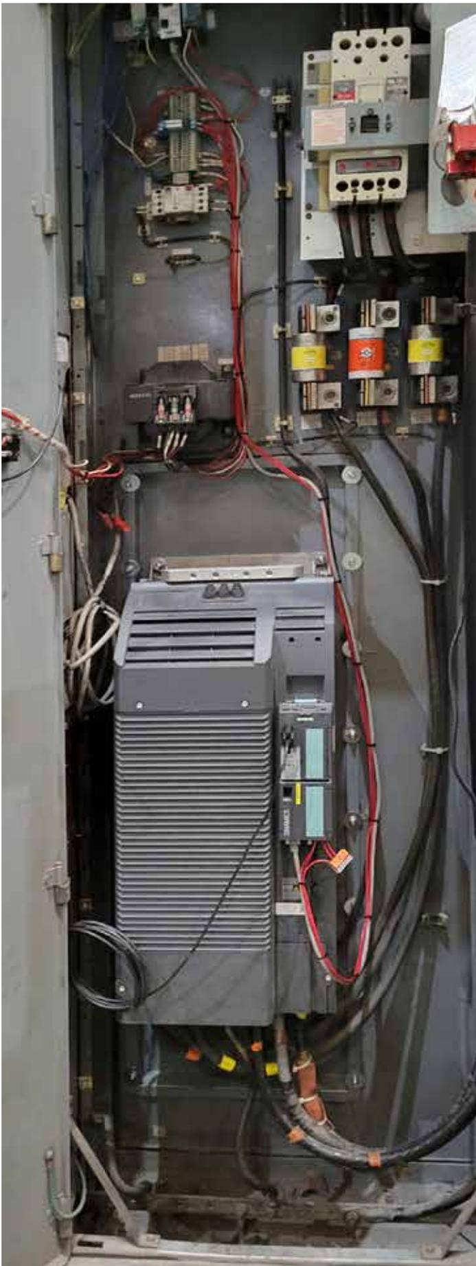
The cooling tunnel fan cabinet with Siemens SINAMICS G120 drive installed.
