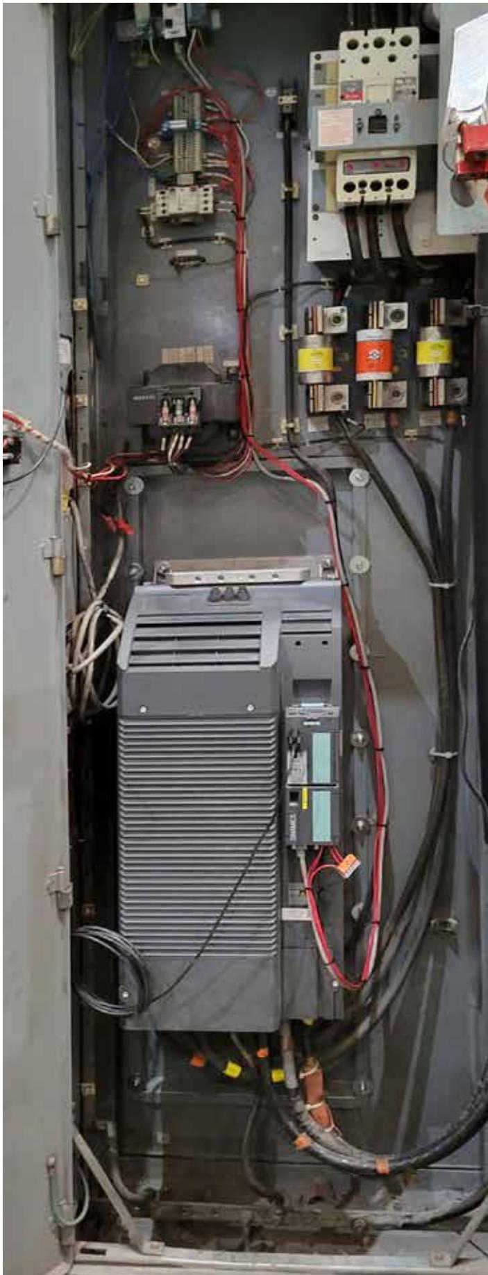
The cooling tunnel fan cabinet with Siemens SINAMICS G120 drive installed.
