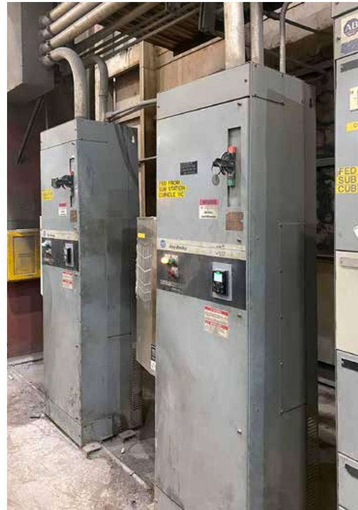
The cooling tunnel 150 hp drives cabinets before conversion. (Courtesy: Century Aluminum)
