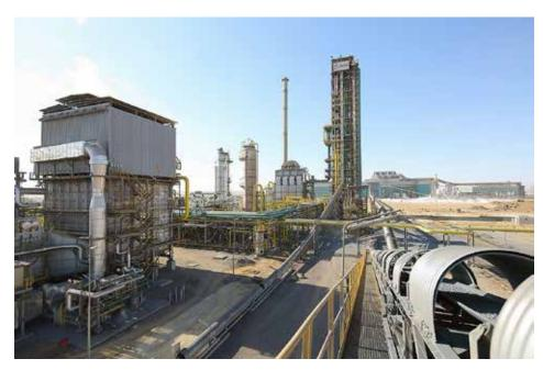
A hydrogen-based 1,000,000 ton/year ENERGIRON® direct reduction plant will reduce carbon dioxide emission. (Courtesy: Tenova)
