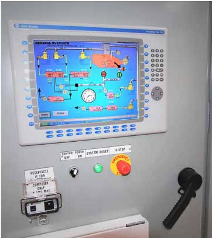
Programmable and user-friendly touch pad controls are essential for operator success and can increase efficiency through variable pre-set parameters. (Courtesy: Epcon Industrial Systems)
