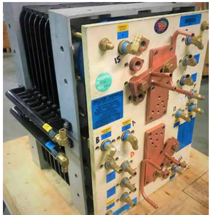
A transformer repair. (Courtesy: Cyprium Induction)
