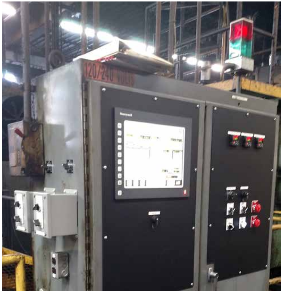
The new system includes an operator interface on the floor for ease of use, and with SpecView software tracking everything, it collects data for anything that records temperatures. (Courtesy: Conrad Kacsik)
