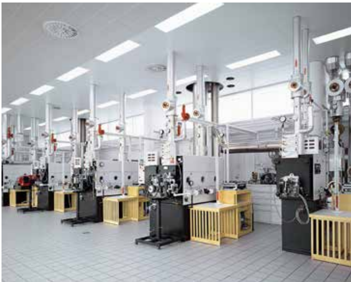
Burner training room.
