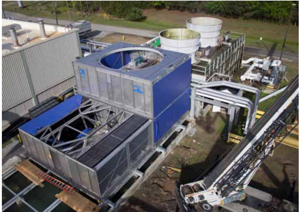
The next generation of factory-assembled cooling towers can be delivered up to 60 percent faster than field-erected towers and installed 80 percent faster. (Courtesy: SPX Cooling Technologies)
